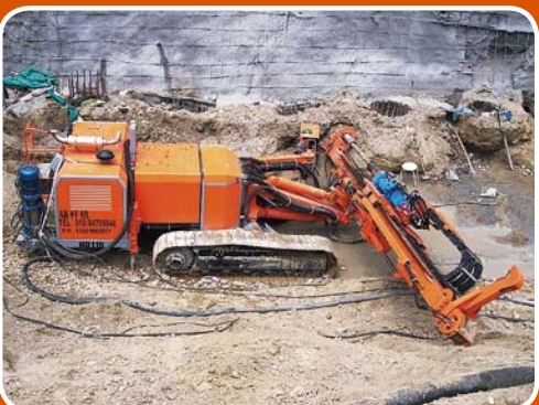
China - Anchor Drilling \phi 133.0\text{mm} China - Ankerbohren \phi 133.0\text{mm}
